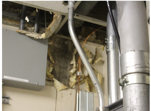
Water penetration and leaks have damaged several parts of the century-old structure. This photo shows some of the water damage in the main electrical room.
